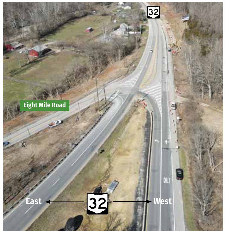
The Eight Mile-State Route 32 intersection will be closed for several months this year.
